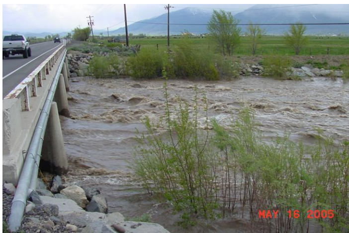
Highway 88 Bridge during 2005 spring run-off
