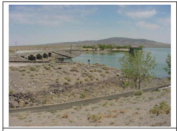
Newlands Irrigation Project Infrastructure – Churchill County, Nevada
